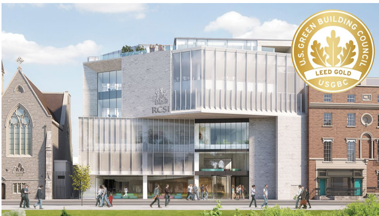
We aim to achieve LEED Platinum and Gold accreditation for both Project Connect and RCSI Connolly Research Centre upon completion in 2024/2025.
